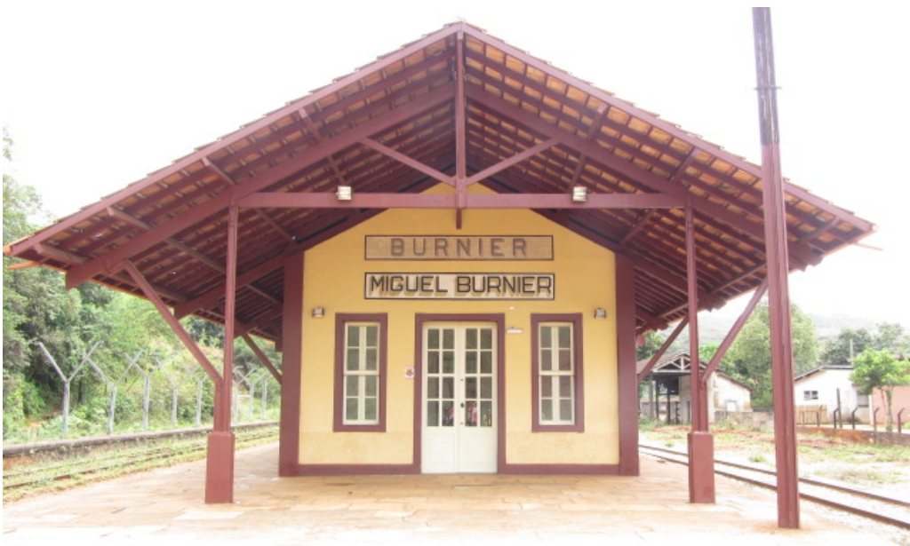
Image 6.2: Miguel Burnier’s train station (restored in 2012), October 4, 2013. Source: own collection
